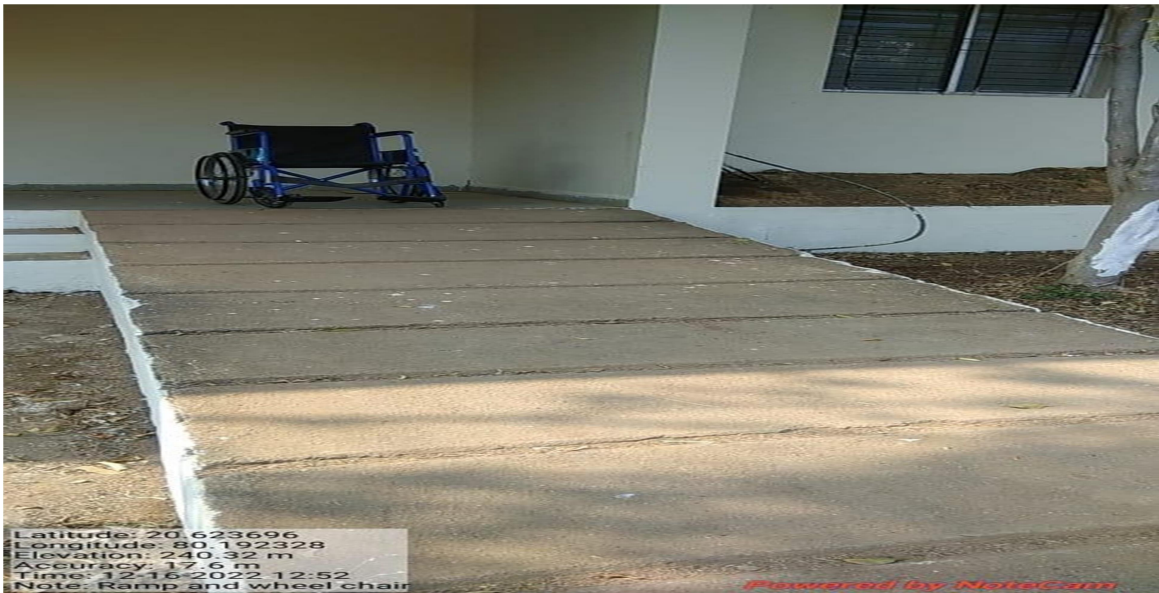
Ramp for Divyangjan
