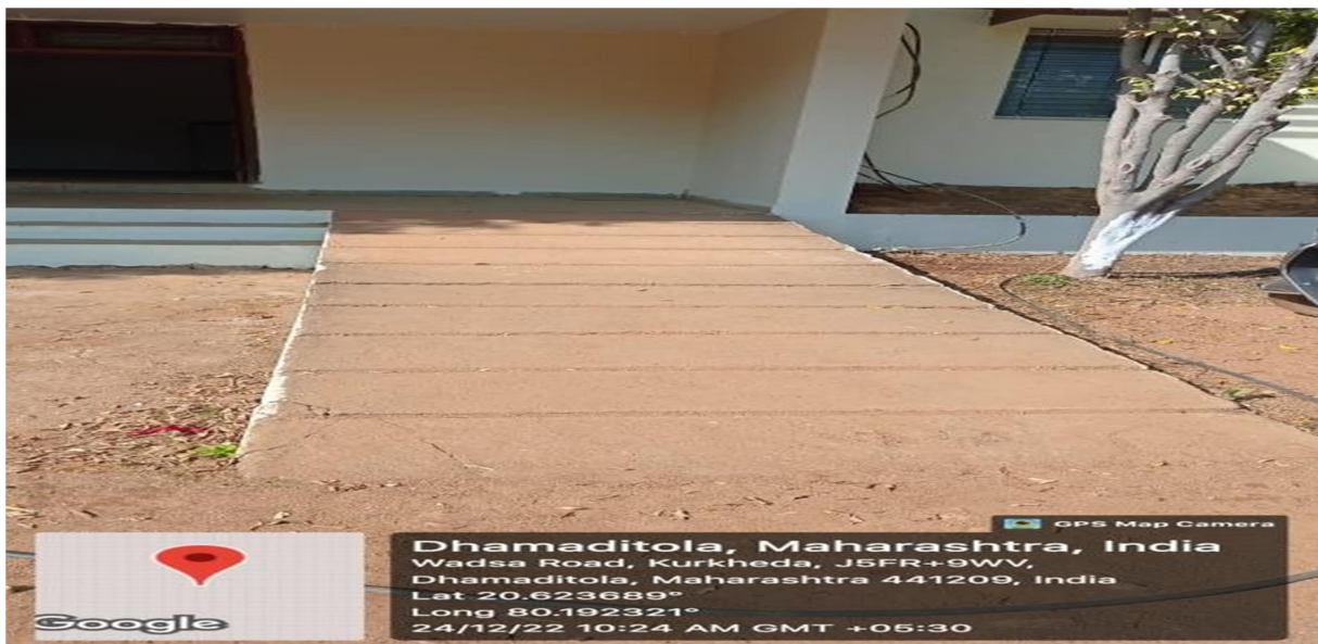
Ramp for Divyangjan
