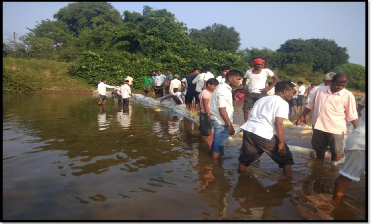
CONSTRUCTION OF POLY-BANDHARA AT SATI RIVER NAWARGAON BY COLLEGE NSS UNIT
